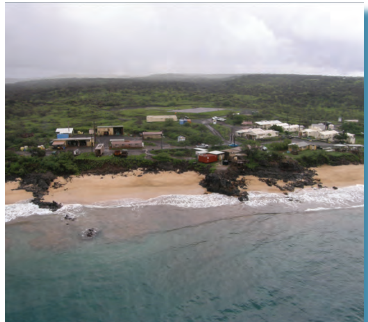
The Honokanai‘a Base Camp, located on the southwestern shores of Kaho‘olawe consist of approximately 22 building and serves as the hub for the volunteer restoration program.
